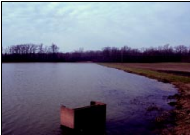
Field at full flood, showing water-control structure.
