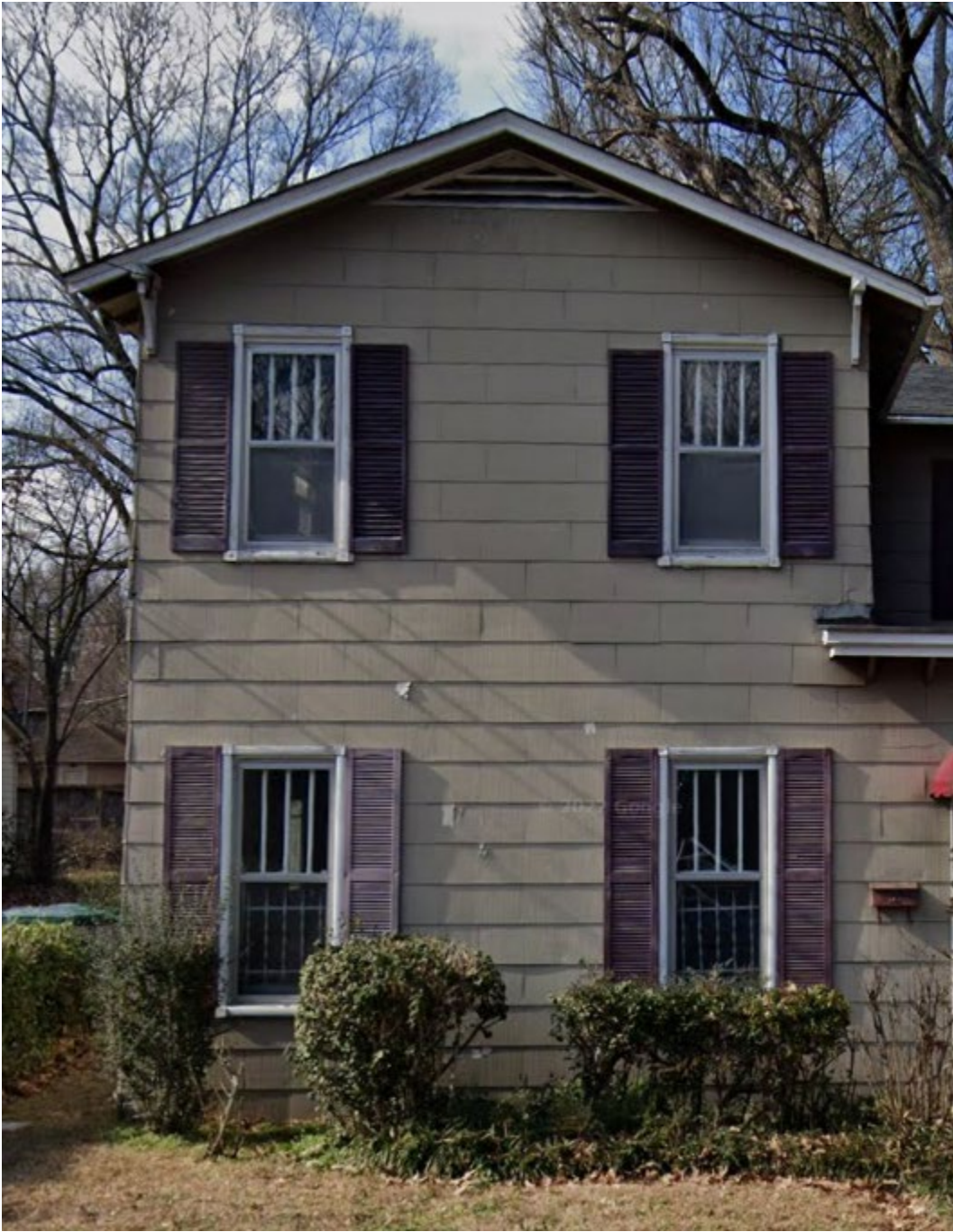
Photo of Original Window Details
